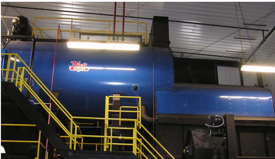
Hurst Boiler & Welding Co., Inc. — Hybrid Super 600 Wood Fired Boiler at Seaman Paper Co.
